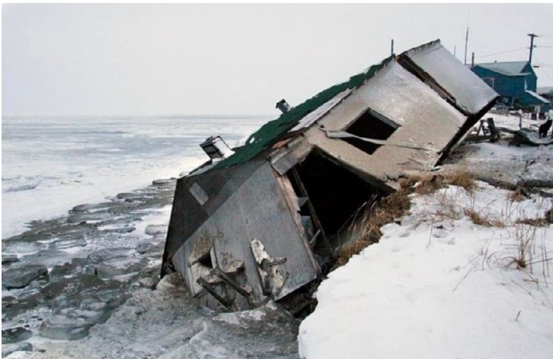
Figure 5. Collapsing buildings as coastal permafrost is thawed and wave action increases, Alaska 17 .
