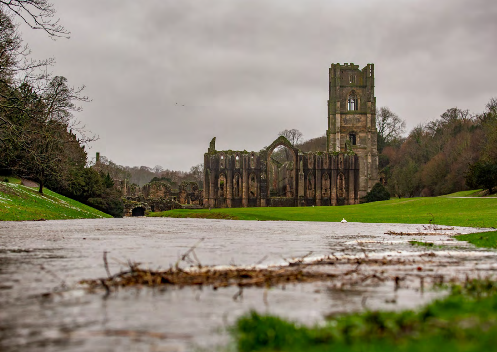
The river Skell breaches its banks on the east green of the abbey at the Fountains Abbey and Studley Royal UNESCO World Heritage Site, UK / National Trust
